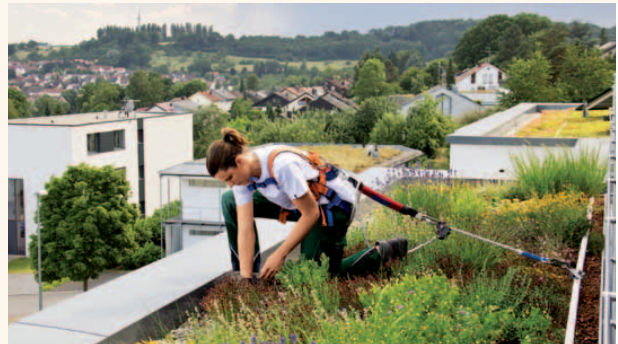
Tried and tested: fall protection systems which do not penetrate the roof
