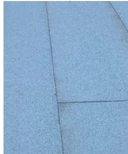
Welded seams on bitumen sheets/welding plastic sheeting
