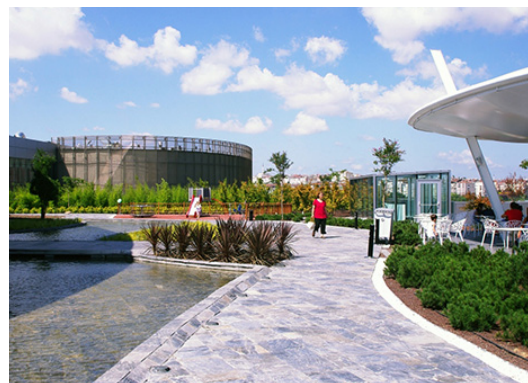
Oase of recreation on the Green Roof of Marmara Forum in Istanbul/Turkey
