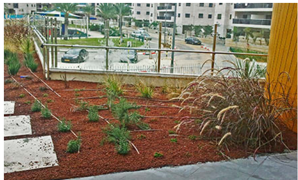
A Green Roof at the Tzuril Elementary School in Rishon Le'Zion was designed with the objective of decorating the environment of the school's second-floor classrooms. Landscape architecture: Zur-Wolf.
