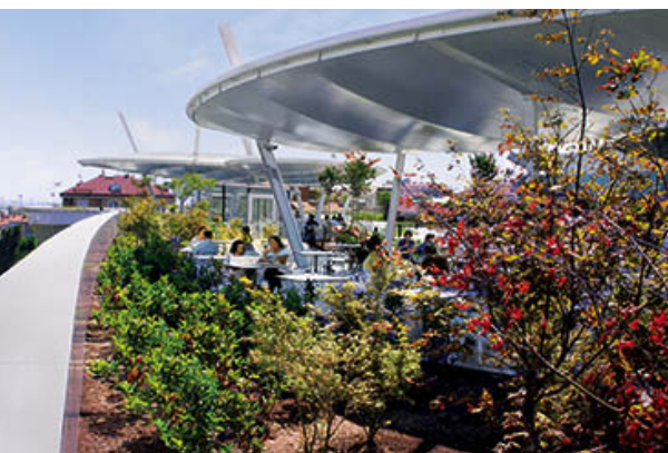
The Green Roof offers a natural atmosphere for the city residents, which is hard to find in the neighbourhood.
