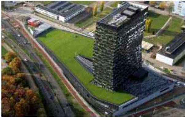
FiftyTwoDegrees (Nijmegen) – Natural stormwater management with green roofs Photo Courtesy IGRA
