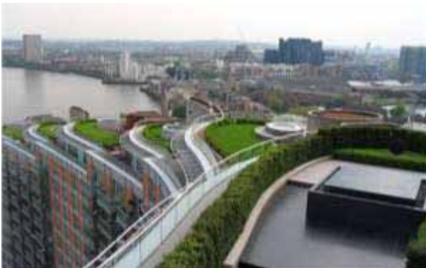
New Providence Wharf (London) – Roof gardens by the Thames Photo Courtesy IGRA
