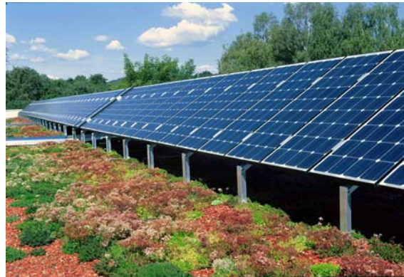
The combination of green roofs and photo voltaic panels offers a lot of synergetic effects (photo: ZinCo GmbH)
